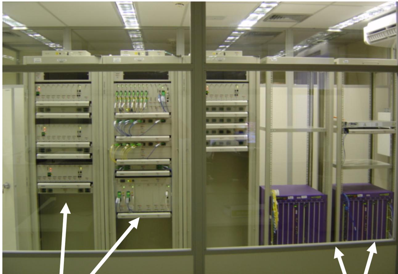
**CPqD DWDM and CWDM Equipment    Extreme Networks L2/L3 Switches**
